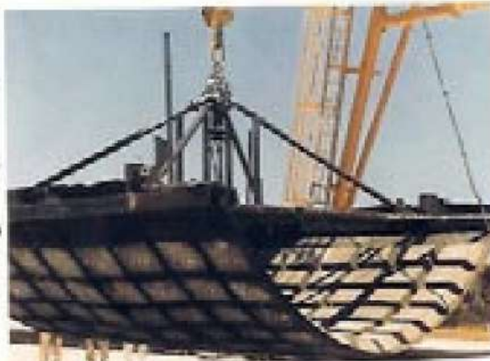
suspended (5 T.) scour control mat before installation at the footing of Woodside Energy's Rankin platform
