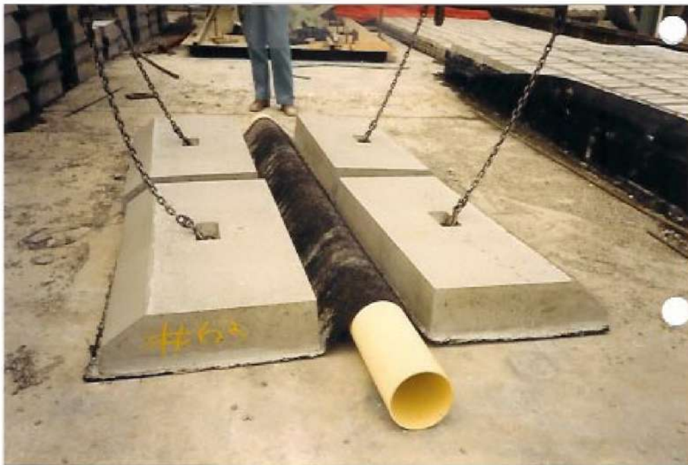
FLEXMAT(S) FOR STABILISATION OF OIL LINE (8") IN CHERVILL FIELD (W.A.)
